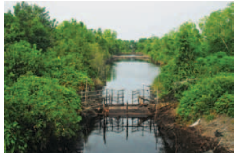
FIGURE 15 Successive ditch blocks made of wood and soil bags in a medium-width canal in Central Kalimantan.
