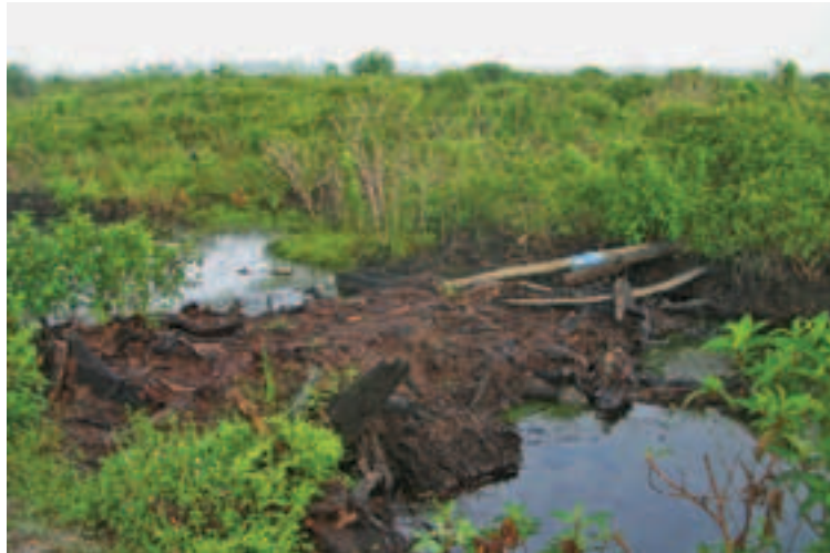
FIGURE 13 Small ditch blocked with peat dam.
