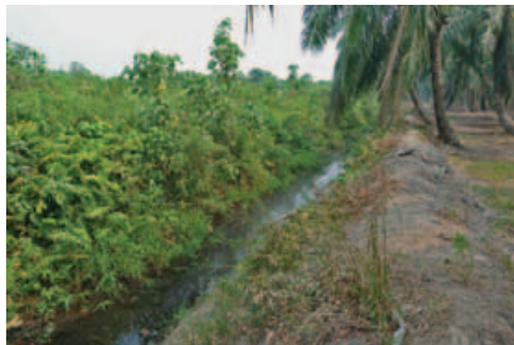
FIGURE 20 Plantation perimeter drain maintained with low water level may lead to drainage of adjacent peat swamp forest thus increasing fire risk.
