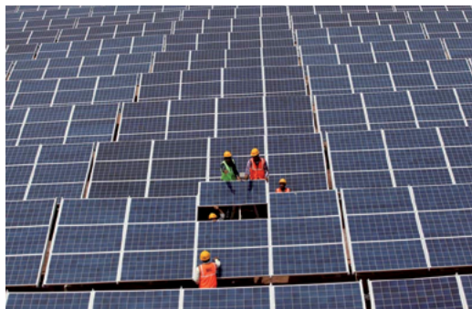
Preparations for the opening of Gujarat Solar Park (Photo credit: DeshGujarat )
