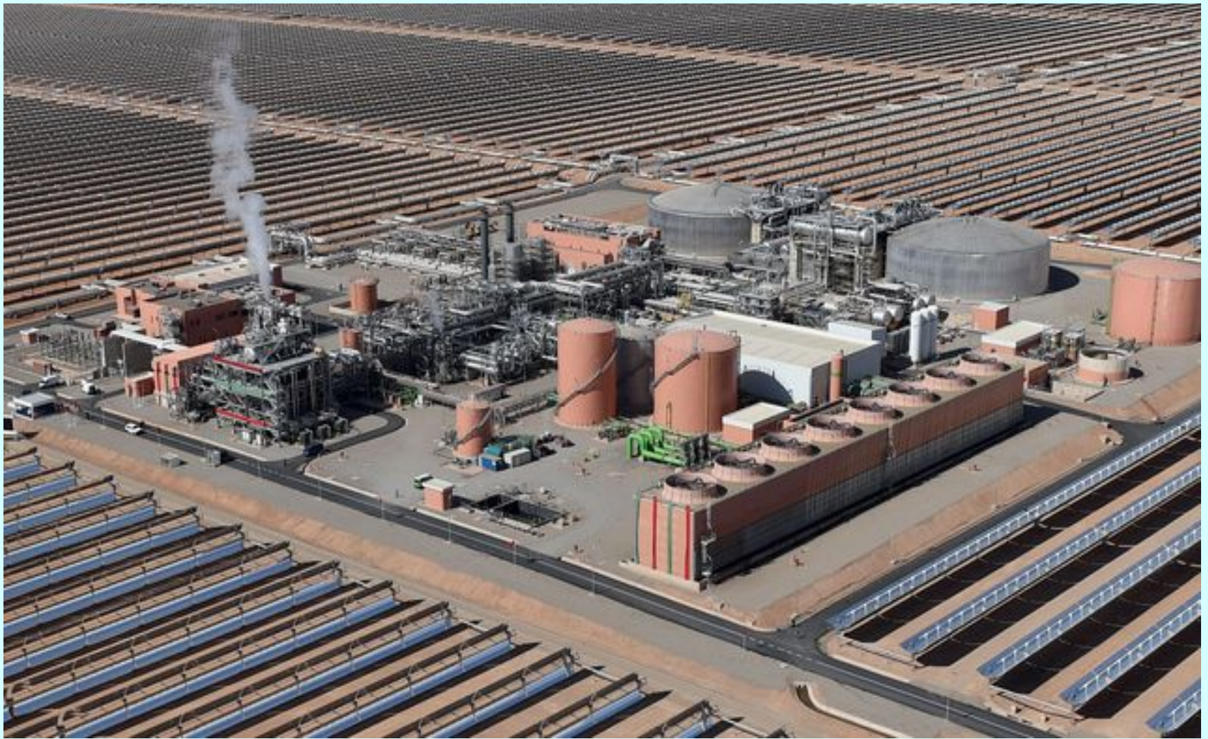
Thermal Solar Power Unit of Ouarzazate (Noor 1, 450 ha)
